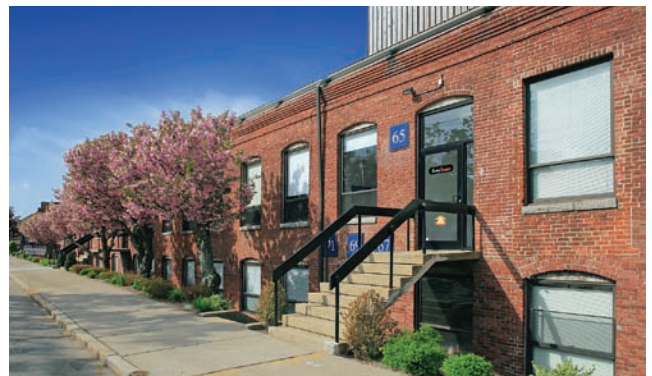
continued on page 42 Chapel Business Center, 59-83 Chapel St., Newton MA
